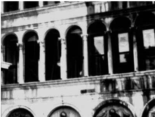
Fig.7. Chemical and abrasive cleaned areas at Piazza San Marco.
